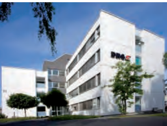
Production Facility, Marburg
